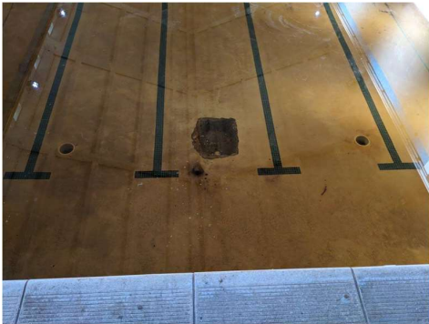
Figure 8- Pool deep end showing hole that requires repair
