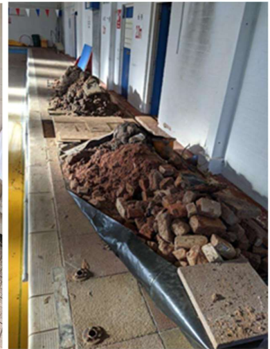
Figure 10- excavations around pool to review filtration system
