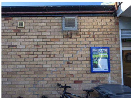
Figure 6- Evidence of masonry cracking Cracking and holes in the pool need to be repaired with waterproofing reinstated where required.
